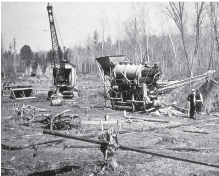
Dragline in operation in the early 1930s, Collins placer gold mine, Goochland County.
